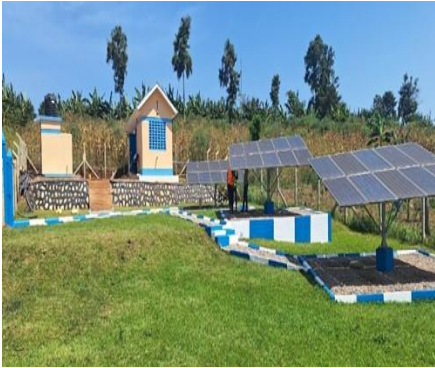
Drinking Water Supply Project in Uganda
